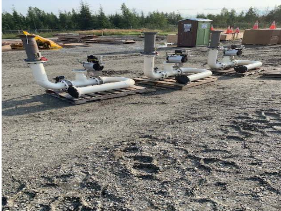
Fabricated Piping for Vaporizer
