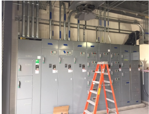
Motor Control Center in Multi-Purpose Building
