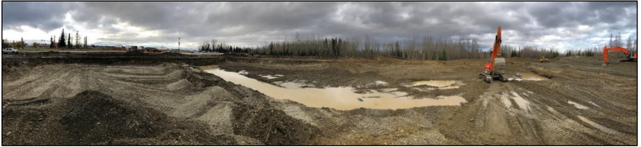
North Pole storage - Ground work preparation for deep dynamic compaction
