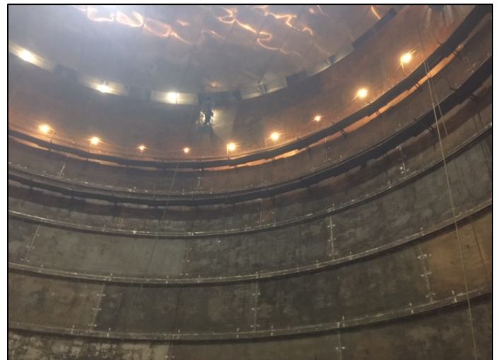
Final inner tank row - Q1 2019
