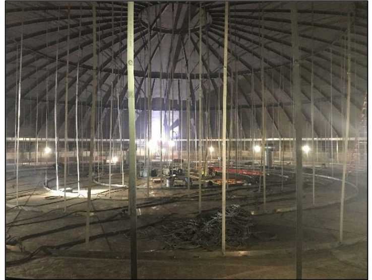
Interior tank suspended ceiling lowered into place – Q1 2019
