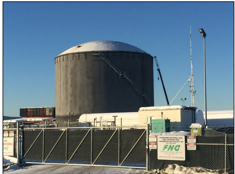
Exterior view of the 5.25 million gallon LNG storage tank - Q1 2019
