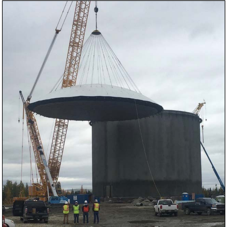
Domed roof weighing more than 120 tons is installed on the LNG tank in September 2018
