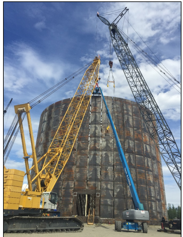
Final panel installation on the 5.25-million-gallon LNG storage tank
